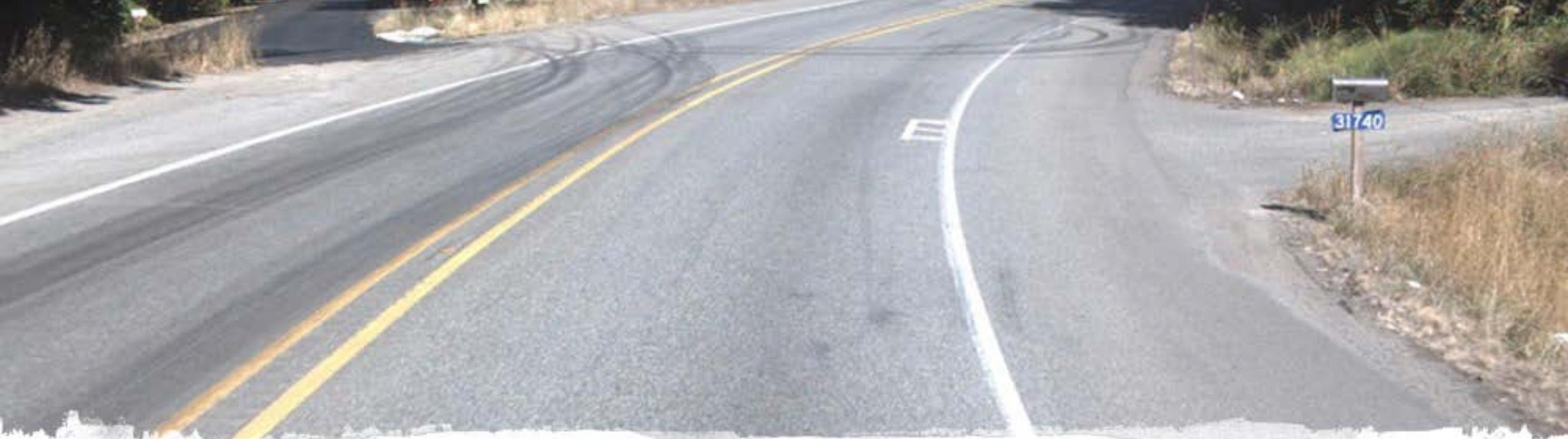
“Because the intensity of the polishing process increases markedly with tread element slip, all other factors being equal, the lowest friction levels are found on high-speed roads, curves, and approaches to intersections; in short, in locations at which high friction values are needed most.”
